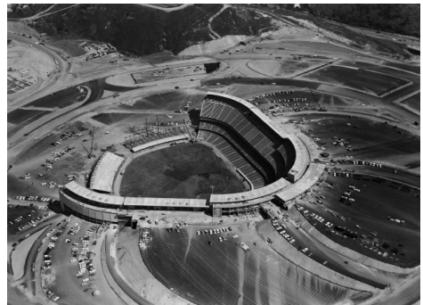
A birds-eye view of the Dodger Stadium construction and terraced parking at Chavez Ravine.
